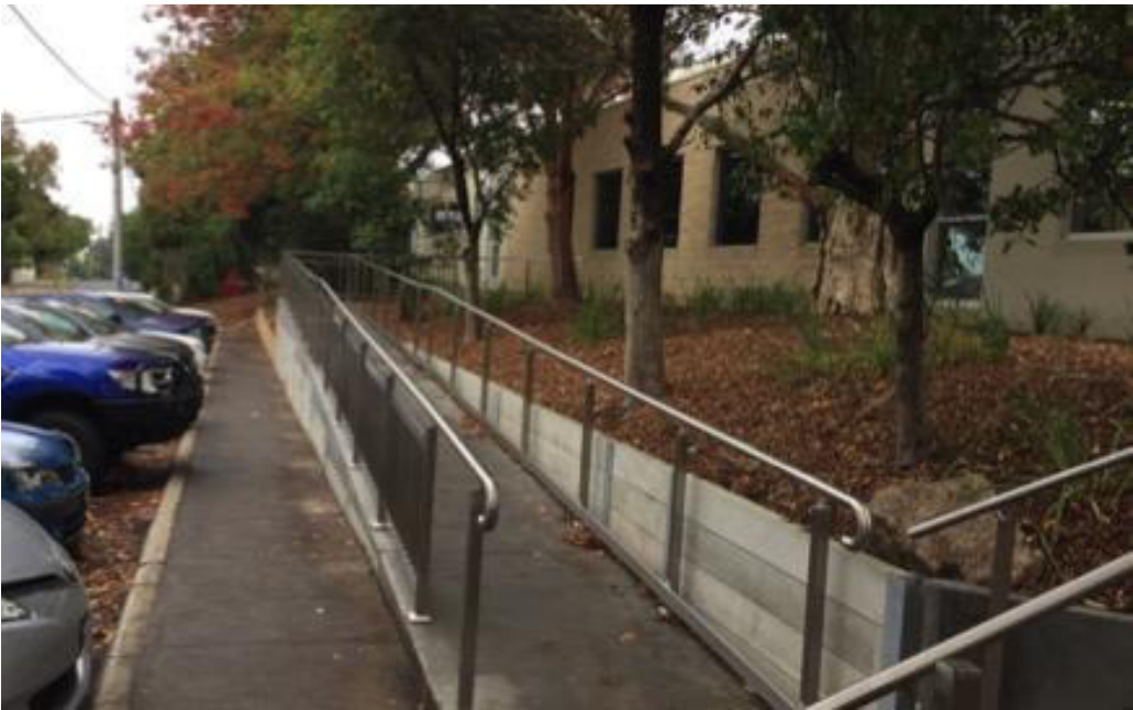
Image 13: Access Ramps and Walkways
